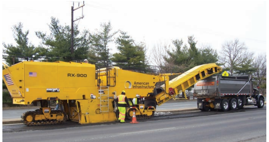
On March 4, Maryland awarded a $2.1-million road resurfacing and improvement project along New Hampshire Avenue in Montgomery County to American Infrastructure. (Photo courtesy American Infrastructure)
